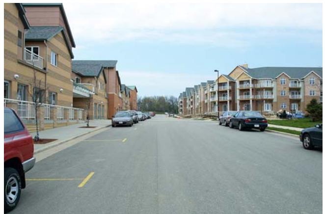
Residential units above commercial space
